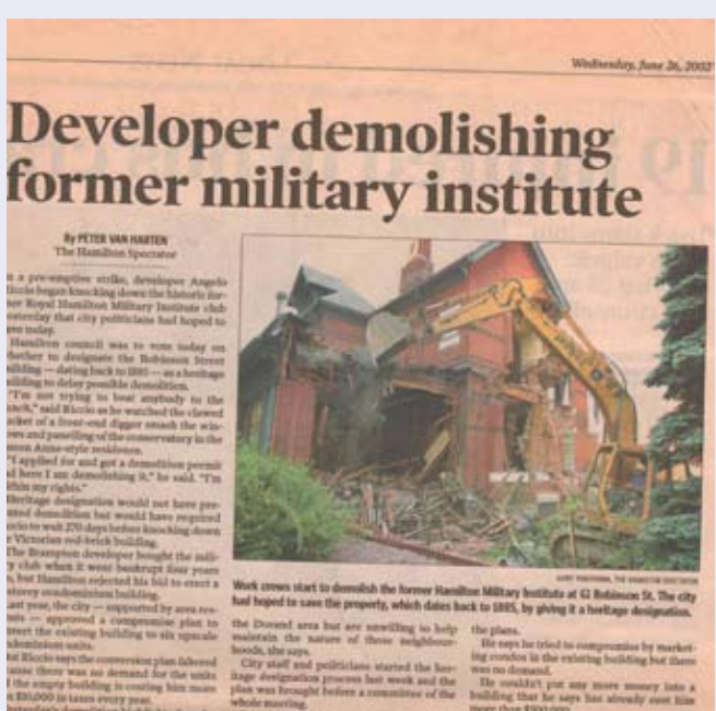
Demolishing Former Military Institute, The Spectator - June 26, 2002
